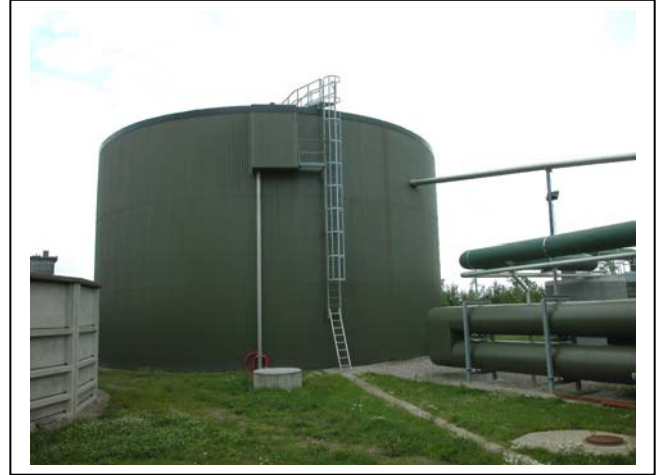
Digester tank and heat exchangers for Pasteurisation
