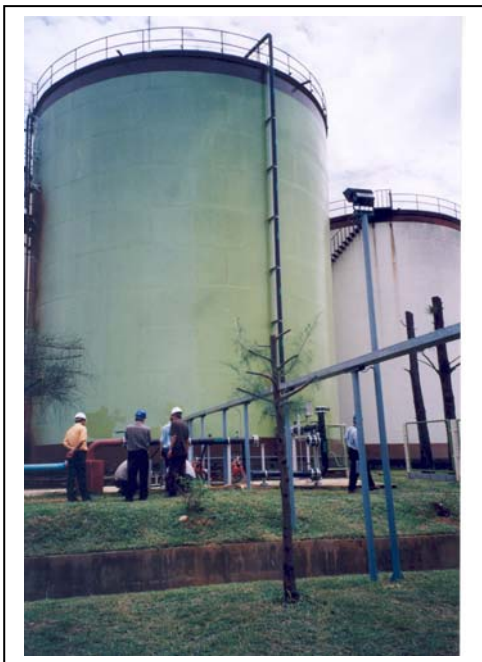
Closed digester tank at an Oil Palm Mill in Krabi
