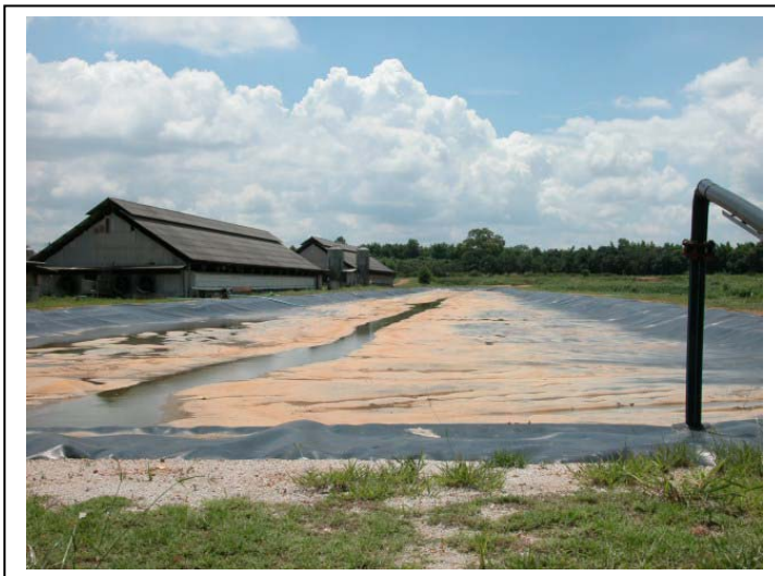
Covered waste water pond at a pig farm in the Chonburi Province
