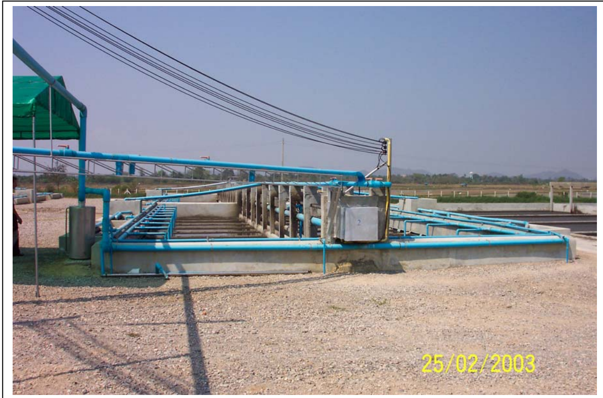
A further developed UASB system called H-UASB (High suspension - Up flow Anaerobic Sludge Blanket) in Ratchaburi
