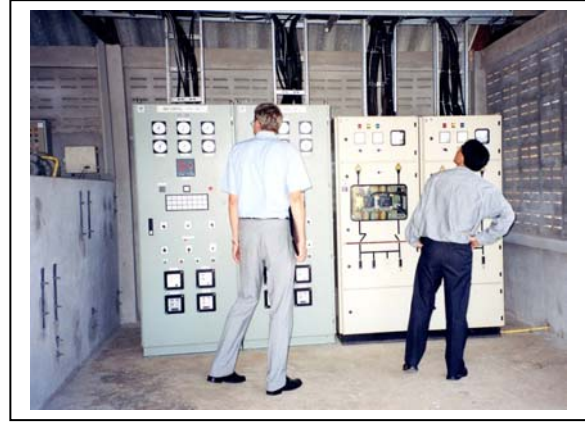
Generator switchboard for electricity supply from the gas engines
