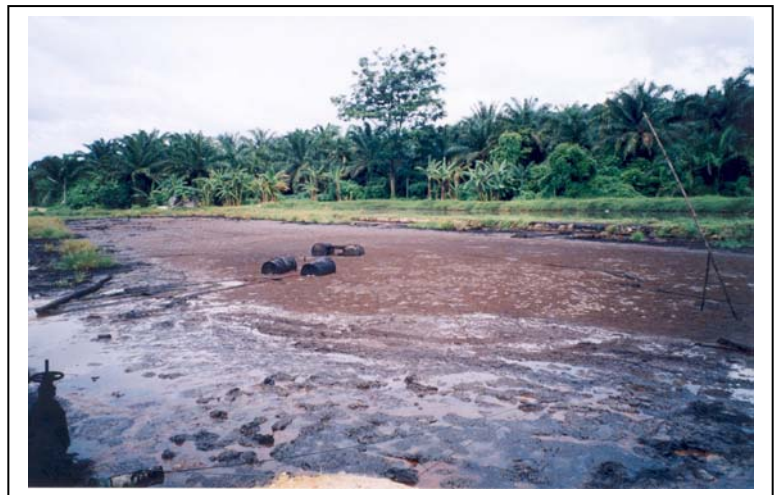
Alternative anaerobic treatment pond at an Oil Palm Mill, where no biogas is collected (Krabi)
