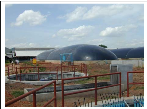
Channel digester, UASB and strainer at a pig farm in Ratchaburi
