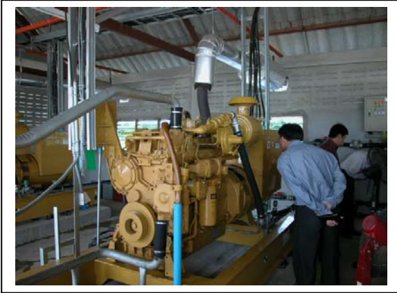
Biogas operated gas engines produce electricity from the gas produced in the cover lagoon in Chonburi
