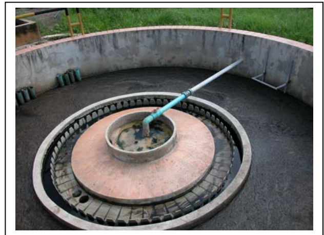
Close up of the top of the UASB and the gas outlet pipe
