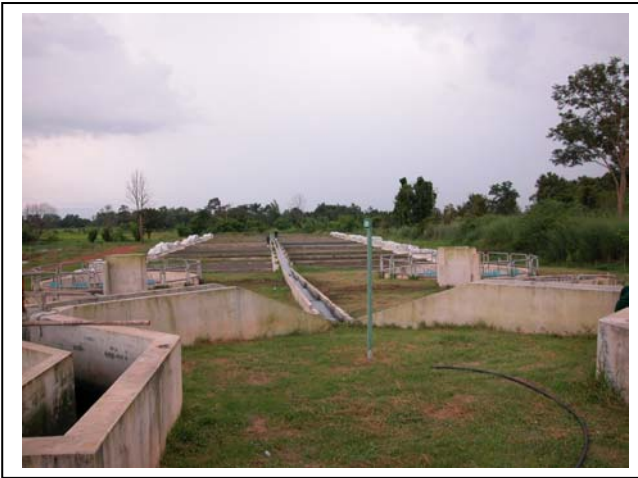
Inlet to the sand bed filter at the pig farm at Ratchaburi
